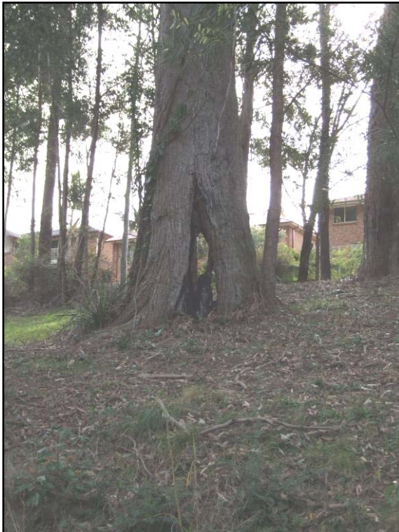
Figure 2 A view of trunk of another tree close to the subject tree Note: the trunk is hollow
